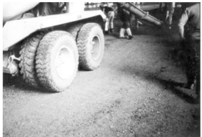
Fig. 4.1.1—Proofrolling by loaded ready mix truck
