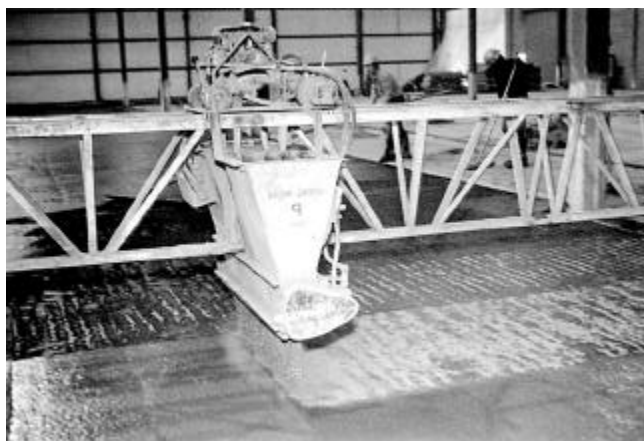
Fig. 8.2.1.2.1—Mechanical spreader FDA, Inc.
