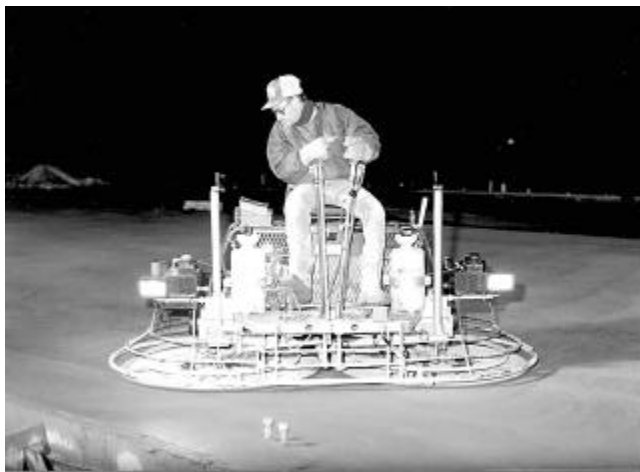
Fig. 8.2.4.4—Double-riding trowel with clip-on pans
