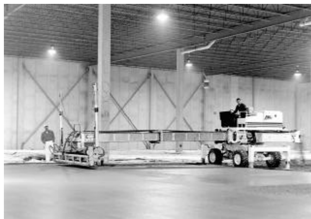
Fig. 8.2.3.2—Laser controlled screed
