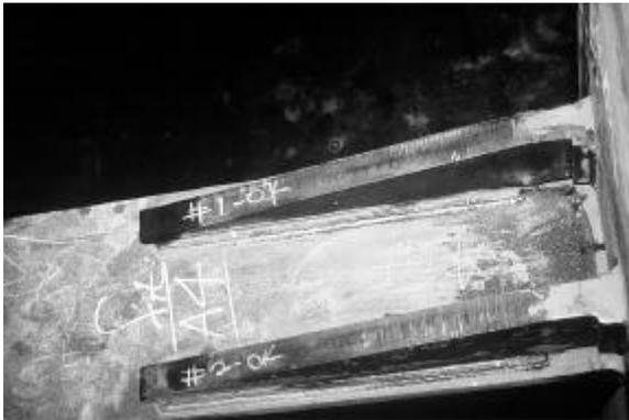
***Connections can be upgraded by welding or bolting new plates onto the beams and columns to change the connection shape and reduce stress concentrations. In some cases, it may also be appropriate to replace defective welds and welds with low toughness with welds with improved toughness and workmanship.***
