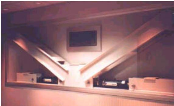
***Energy dissipation systems are typically installed in buildings as part of a vertical bracing system that extends between the building's floors.***
