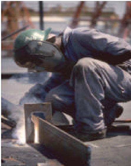
***If inadequately constructed, welded joints in moment-frames can be weak links that fail prematurely. FEMA 350 recommends careful control of the materials, workmanship and procedures used to make these joints and verify their adequacy.***
