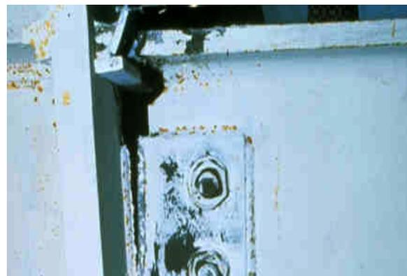
**Fracturing of welded connections can lead to damage to the bolted connections that hold the beams onto the columns, creating potential for localized collapse.**
