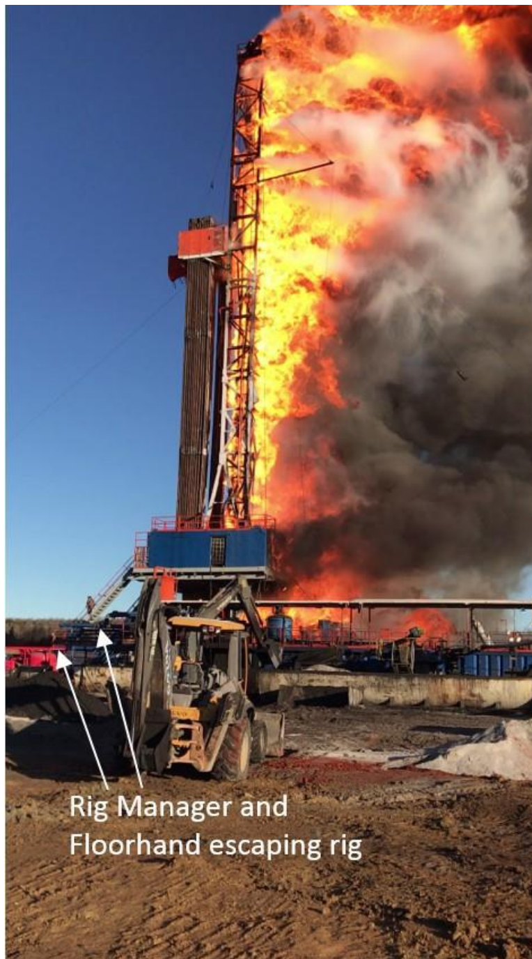
Figure 43. Still from video captured at 8:36 am, shortly after blowout started. The rig manager and floorhand can be seen escaping the rig. At this point, the fire has engulfed the driller's cabin (far side of photo).
