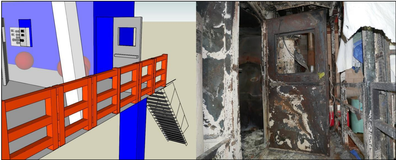
Figure 46. The most viable exit door was hinged such that when the door was opened, the door blocked the escape path to the ground.
