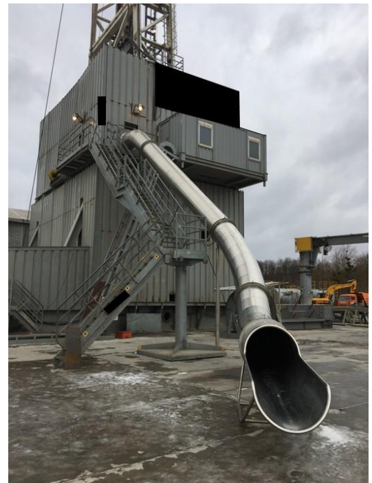
Figure 47. Example design strategy to provide quick egress from drilling rig during a blowout.
