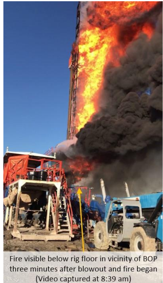
Figure A- 6. Video still of Patterson Rig 219 fire, taken 3 minutes after blowout began.
