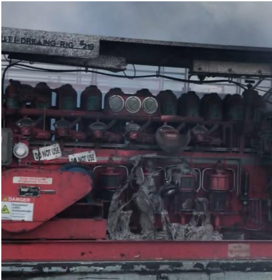
Figure 32. Video captured at 11:51 am on January 22, 2018 shows all BOP handles in the closed position.
