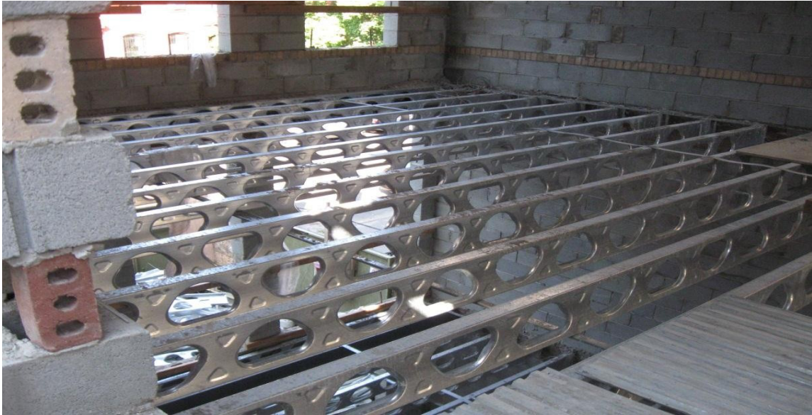
Fig. 6 Floor joists spaced at 16" o/c.
