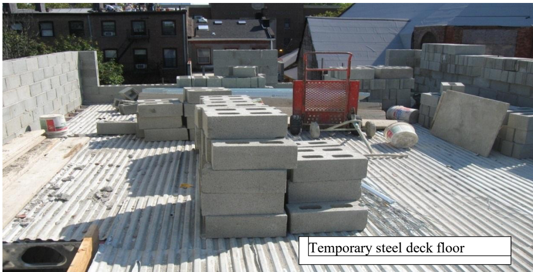
Fig. 7 Temporary steel deck on 225 Carlton Ave. supporting construction loads.
