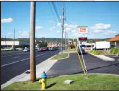
Multiple driveways create potential conflict points for bicycles, pedestrians and motor vehicles.
