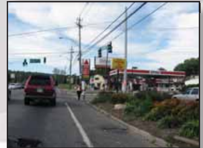
Missing or inadequate sidewalks make walking difficult, unsafe, and in some cases, impossible.
