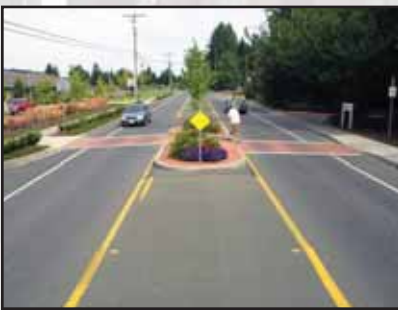
A 'Z' configuration causes pedestrians to face oncoming traffic at mid-block crossing locations.
