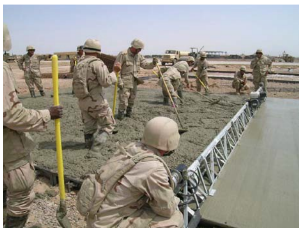
Figure 66 – Mechanical screed.
