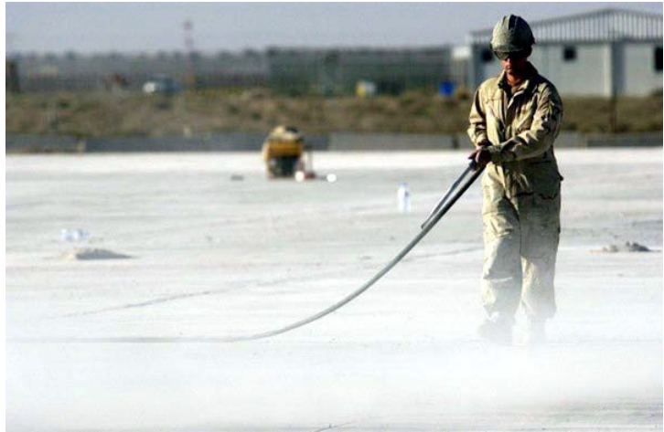
Figure 78 – Sprinkling concrete with water.
