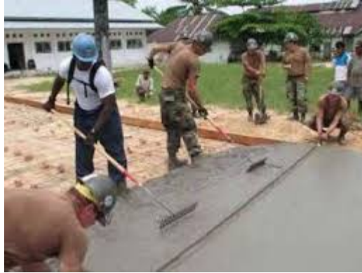
Figure 67 – Concrete placement.
