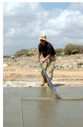
Figure 71 – Long handled float in use.
