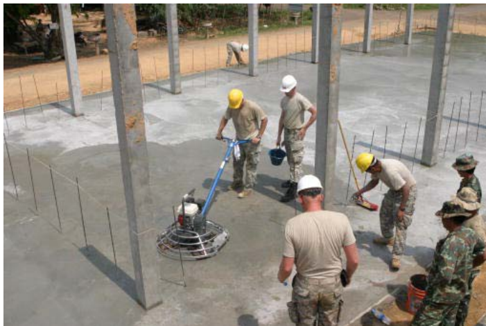
Figure 6-76 – Mechanical troweling machine.
