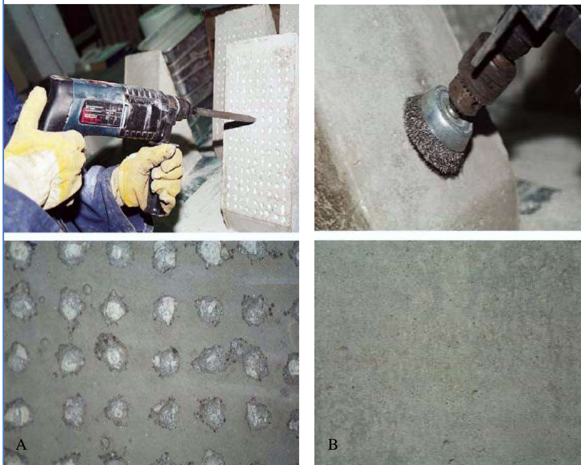
Figure 3.2. A) Substrate surface partially chipped, B) Substrate surface prepared with steel brush (Julio et al., 2004)
