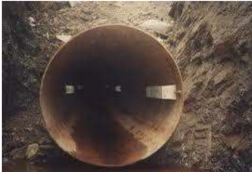
Fig. 10, Internal cathodic protection of pipeline by sacrificial anode method
