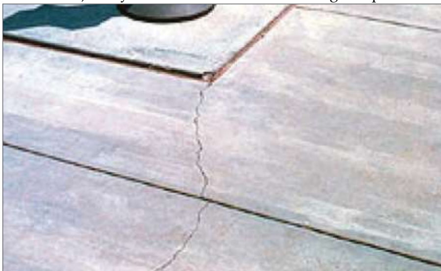
Figure 3. Drying Shrinkage Cracking.
