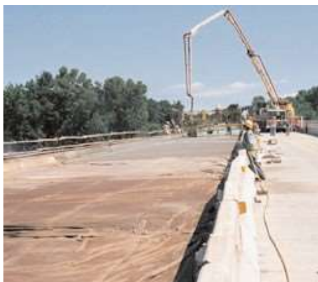
Fig. 12-1. Curing should begin as soon as the concrete stiffens enough to prevent marring or erosion of the surface. Burlap sprayed with water is an effective method for moist curing. (69973)
