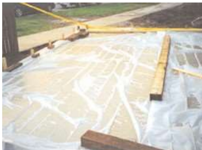
Fig. 12-7. Polyethylene film is an effective moisture barrier for curing concrete and easily applied to complex as well as simple shapes. To minimize discoloration, the film should be kept as flat as possible on the concrete surface. (70014)
