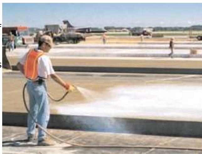
Fig. 12-8. Liquid membrane-forming curing compounds should be applied with uniform and adequate coverage over the entire surface and edges for effective, extended curing of concrete. (69975)
