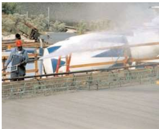
Fig. 12-4. Fogging minimizes moisture loss during and after placing and finishing of concrete. (69974)
