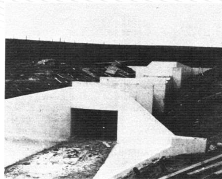
Figure 4-21. Concrete box culvert with concrete percolation collars. P328-701-3743
