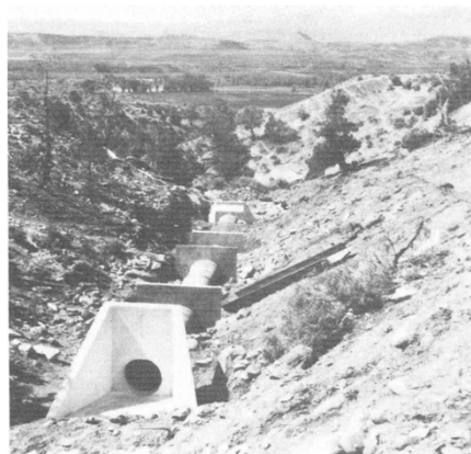
Figure 4-19. Culvert, constructed prior to construction of canal. P514-417-366
