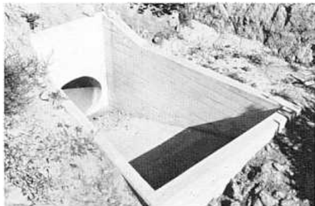
Figure 7-7. Type 4 inlet concrete transition. P-328-701-9300
