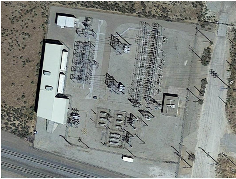
Figure 4. A monolith substation and BESS facility in Tehachapi, California. The BESS provides transmission services, system capacity, and ancillary services.
