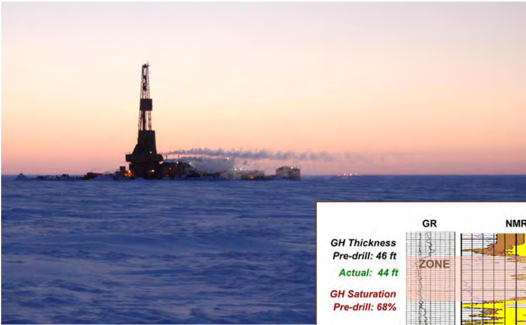
Logs from Mt. Elbert test well in Milne Point field near Prudhoe Bay on the Alaskan North Slope. The gamma ray (GR) and nuclear magnetic resonance (NMR) logs show that pre-drilling estimates of formation thickness and methane hydrate gas saturation (Sgh) based on seismic data were very accurate, supporting the conclusion that seismic exploration tools could be used to prospect for methane hydrate deposits. (Courtesy of Mt. Elbert Science Team)
