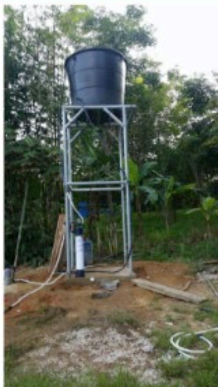
Fig. 1: Install water storage tanks with RFU*
