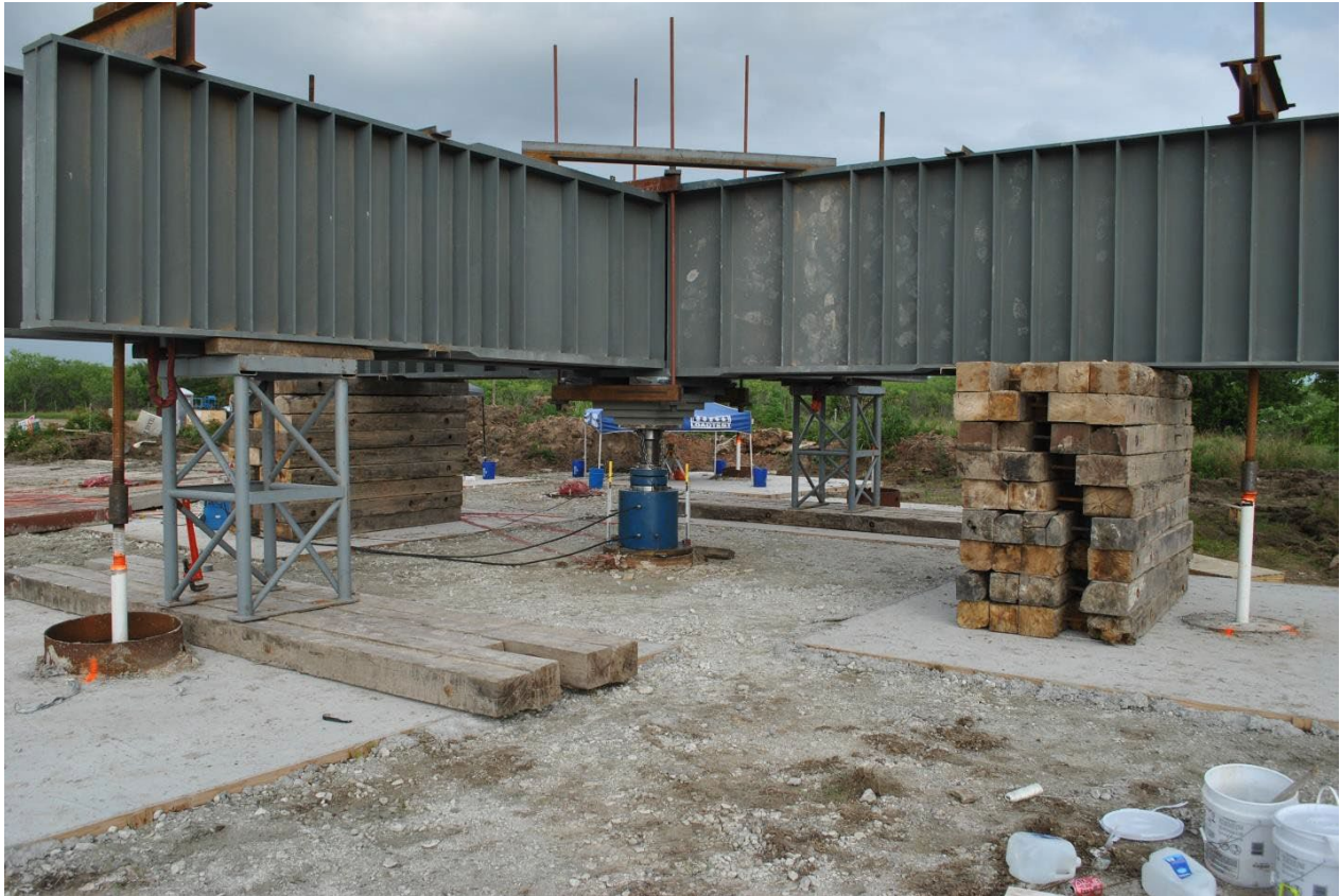
Figure 10.7: Load test setup for top-down loading.
