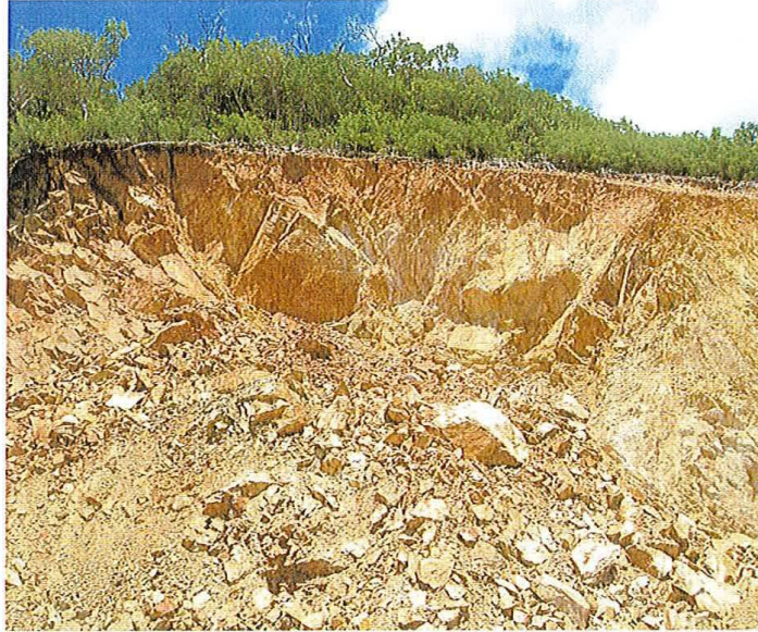
Figure 17. Upper Portion of the Collapsed Surface (Center), Looking Toward West.
