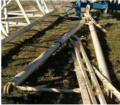
The First Failure
