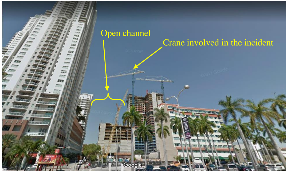
Figure 17 Street view of the first failure site – looking west* (Courtesy of Google Map, May 2017)
