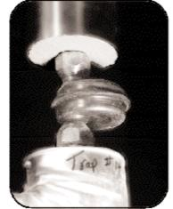
inside the trap when the steam system is shut down. Replace traps subject to freeze damage with self-draining types.
