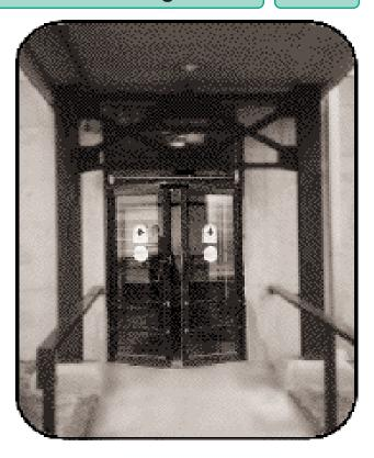
Properly placed automatic doors and vestibules can reduce unwanted air leakage in buildings. Ensure the outdoor areas where people congregate, such as smoking areas, are not within electronic "view" of the automatic controls.
