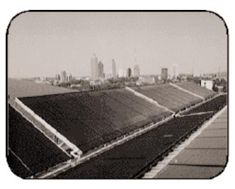
Solar thermal water heating can meet hot water demand at very low operating cost. Flat plate collectors are in the middle of the photo. Also shown are PV panels on the flat portion of the roof.
