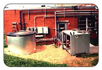
Thermal storage on HVAC systems is effective at cutting peak electrical demand.
