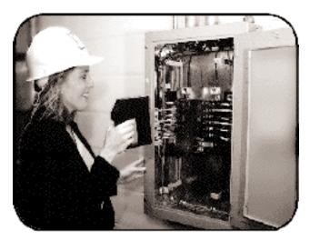
Infrared thermography can quickly identify electrical power system problems and should be included in a proactive maintenance program.
