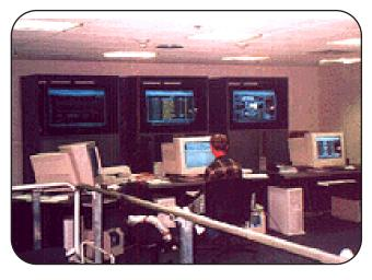
Energy Management and Control Systems can monitor and control equipment throughout a facility from a single location.
