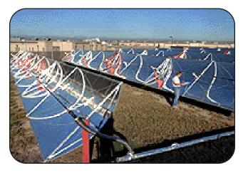
Solar water heating is a proven technology that directly substitutes renewable energy for conventional water heating. This array of parabolic trough collectors was paid for through an Energy Savings Performance Contract (ESPC).
