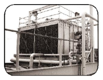
Cooling towers, which are usually components of large HVAC systems, can be made more efficient by controlling their operation times and by retrofitting their motors with variable frequency drives.
