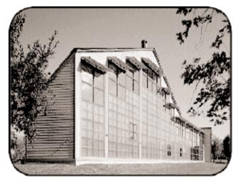
This passive solar building incorporates trombe walls, daylighting, and awnings.
