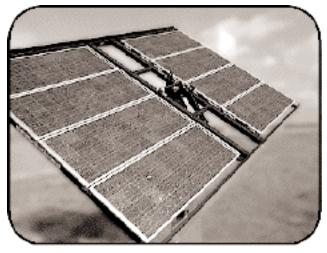
Photovoltaic panels are frequently mounted on devices that track the sun.
