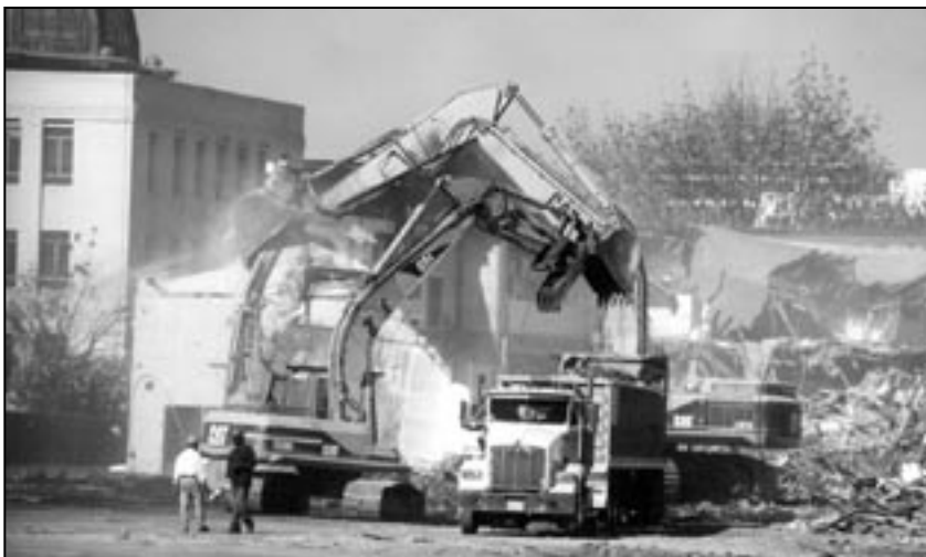
Photo: RecycleWorks Green Building Program
