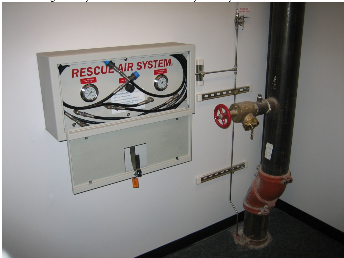
Figure 16.2 - Fire fighter air refilling station located inside a stairway Photo by Joe McElvaney
