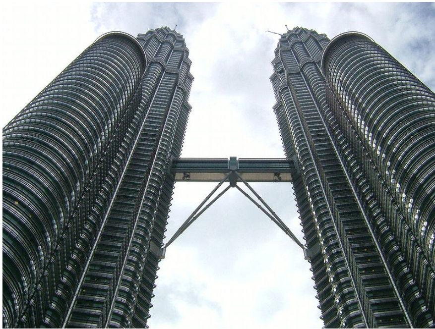
Figure 10.1 – The sky bridge connecting the two towers of the Petronas building in Kuala Lumpur which is used for the horizontal transfer of occupants between the towers in a fire condition
