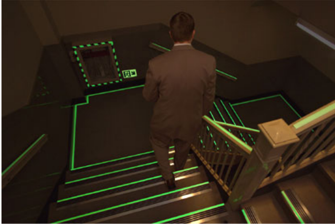
Figure 10.4 – Egress stairway provided with photoluminescent markings Photo courtesy Balco, Inc.
