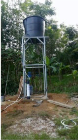
Fig. 1: Install water storage tanks with RFU*
