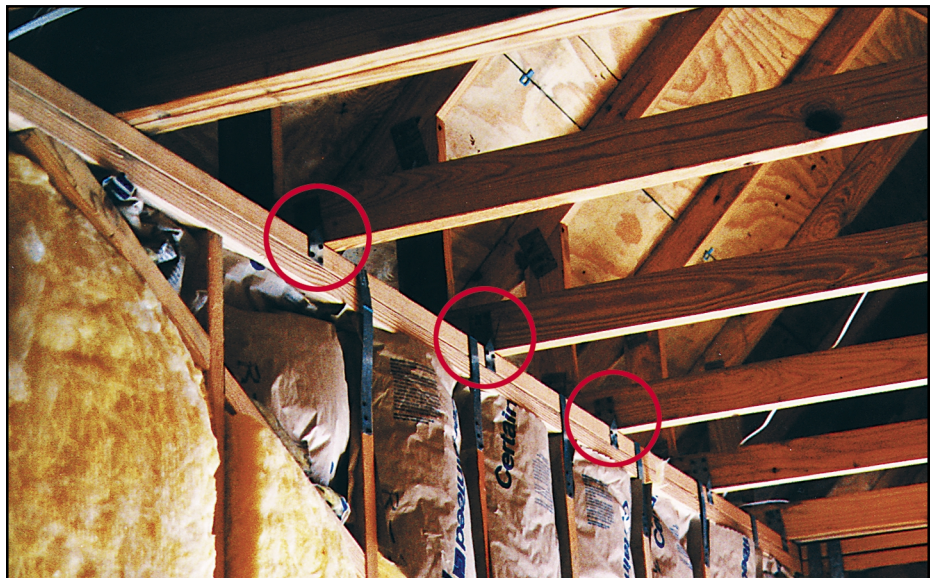
Figure 12-35 Typical connection of truss to wood wall.
