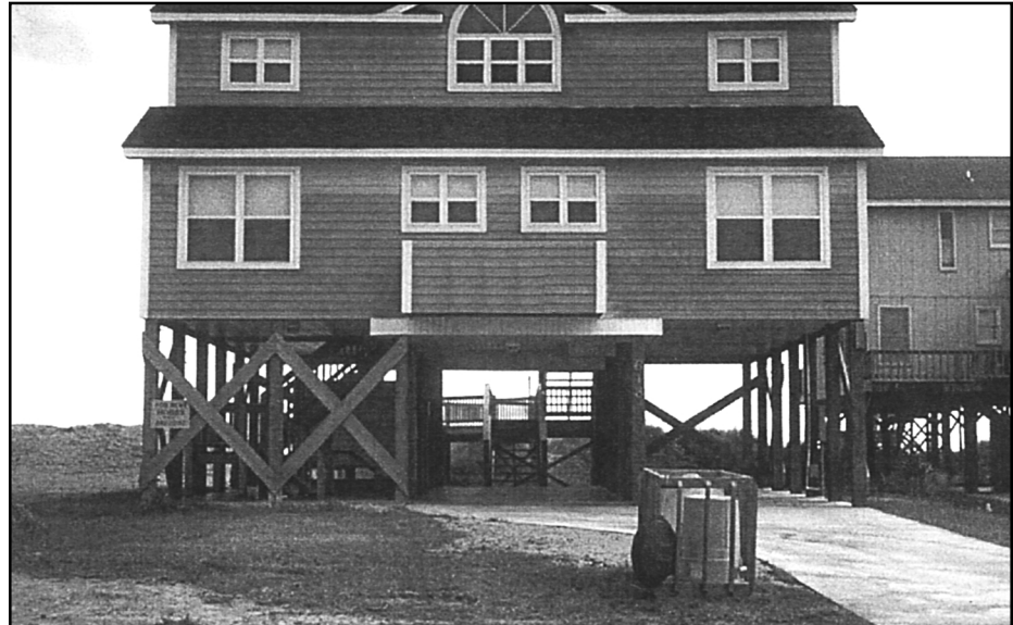
Figure 13-8 Diagonal wood bracing in a wood-pile foundation.
