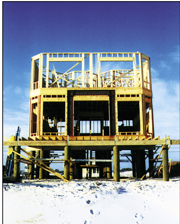
Figure 12-49 Steel moment frame at large opening.
