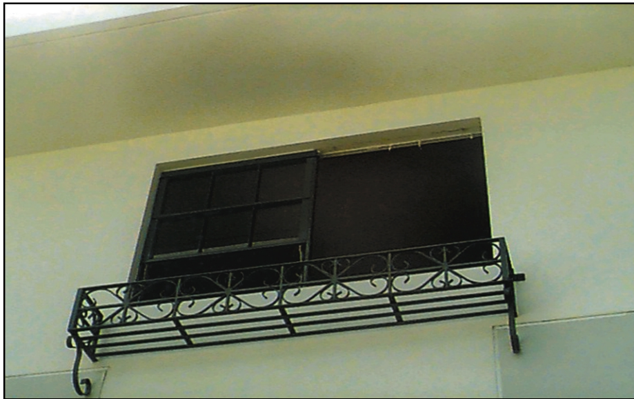
Figure 12-92 Hurricane Georges (1998), Puerto Rico. Inadequate window frame attachment caused the window frame to be pulled out of the wall.
