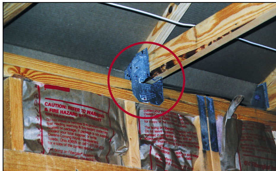
Figure 12-36 Typical connection of truss to wood wall.
