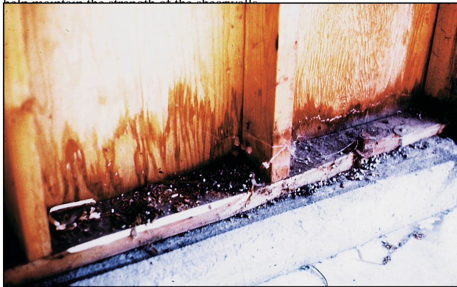
Figure 14-5 Deteriorated wood sill plate.
