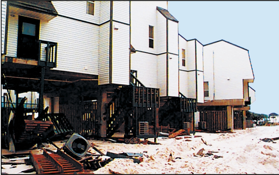
Figure 12-114 Hurricane Georges (1998), U.S. Gulf Coast. Mechanical equipment damaged as a result of insufficient elevation.
