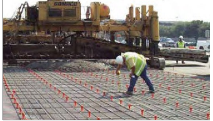
Figure 61. Checking for position and movement of longitudinal steel.
