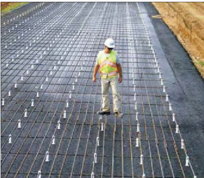
Figure 30. Worker inspecting longitudinal reinforcing steel with transverse bars and chairs (Virginia).
