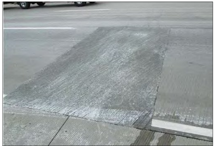
Figure 72. Completed FDR in CRCP.
