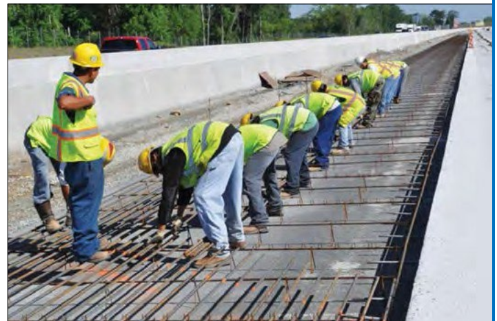
Figure 35. Placing longitudinal steel on TBAs.
