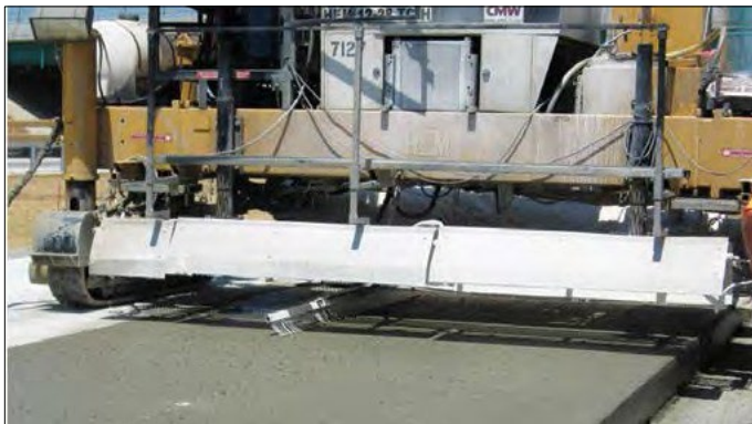
Figure 39. Applying transverse tining on a new CRCP.
