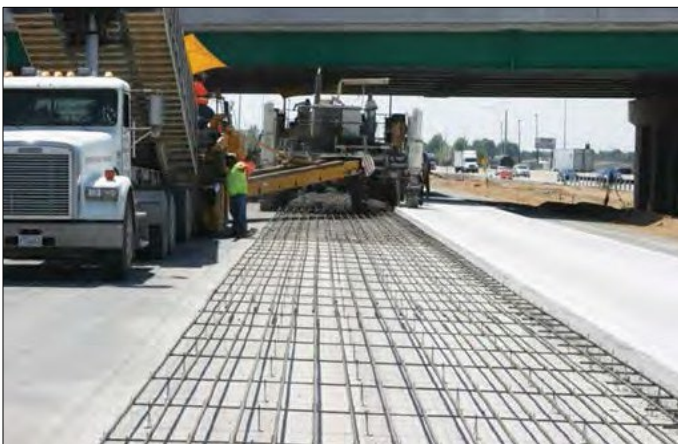
Figure 77. Unbonded CRCP overlay under construction.
