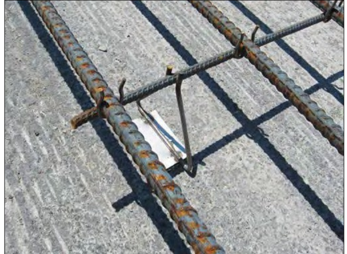
Figure 34. Transverse bar assembly (TBA).
