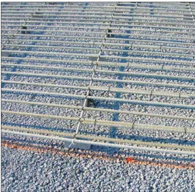
Figure 65. GFRP longitudinal reinforcement for CRCP (Canada).
