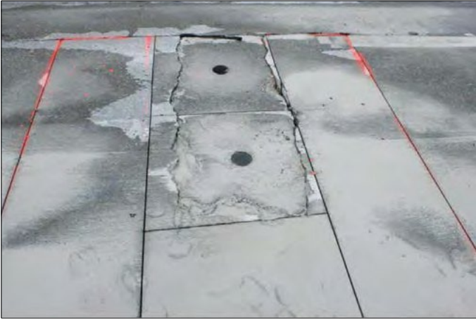
Figure 69. Full-depth and partial-depth saw-cuts at boundaries of CRCP repair area.
