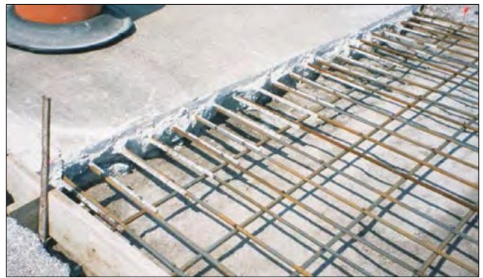
Figure 71. New steel in FDR spliced to longitudinal steel exposed in CRCP.
