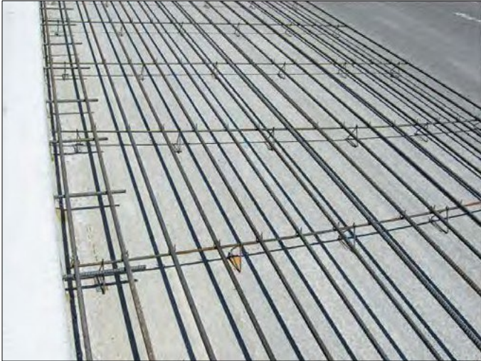
Figure 33. Steel placed on transverse bars assemblies (Illinois).
