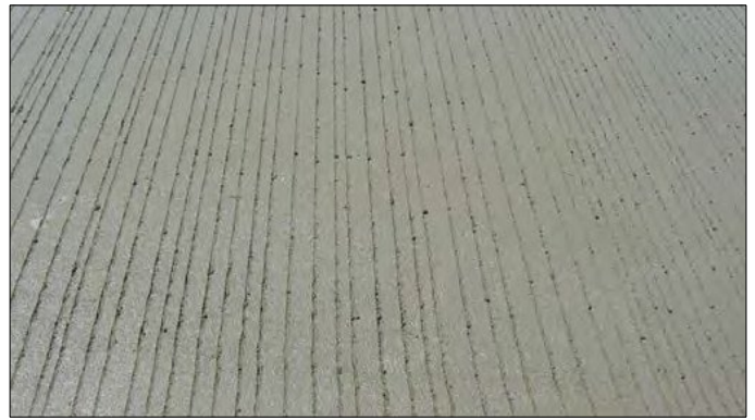
Figure 40. Transversely tined fresh concrete on a new CRCP.
