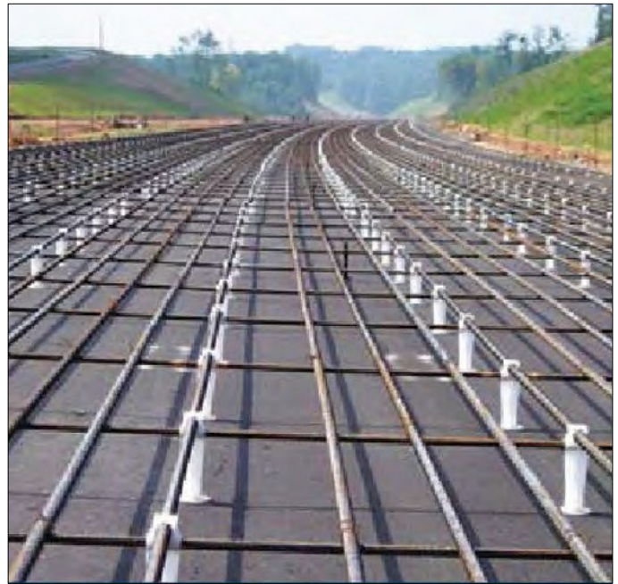
Figure 22. Steel placed on ATB (Virginia).
