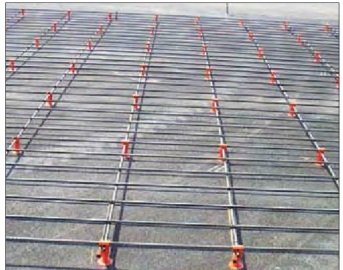
Figure 31. Steel placed on chairs (Texas).
