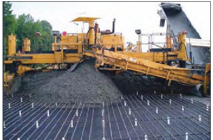
Figure 4. Concrete mixture design and materials are critical for good performance.
