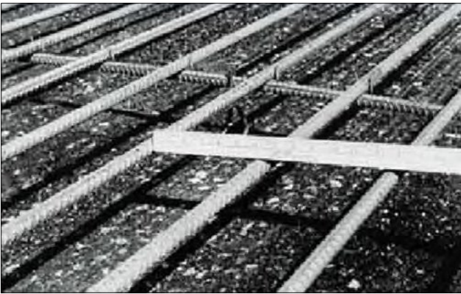
Figure 60. Lateral spacing of longitudinal steel.
