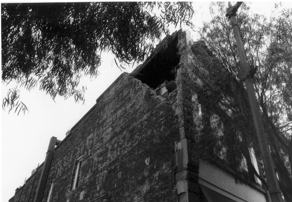
**Figure 7-12** Photo of Corner Damage (from Rutherford and Chekene, 1990)
