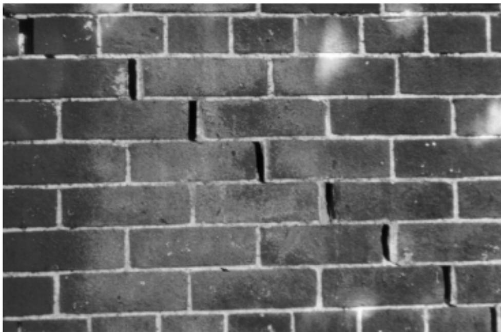
**Figure 7-10** Photo of Bed Joint Sliding
