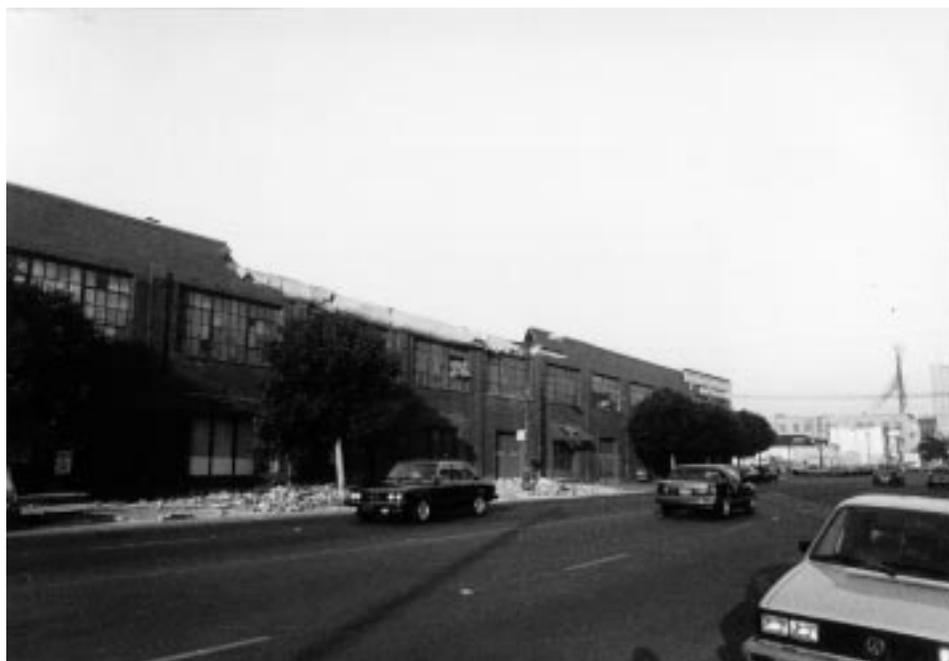
**Figure 7-2** Photo of Parapet Failure (from Rutherford and Chekene, 1990).
