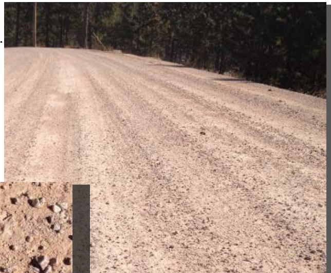
High quality surface gravel with a good blend of stone, sand and fine-sized particles on a mountain road.
