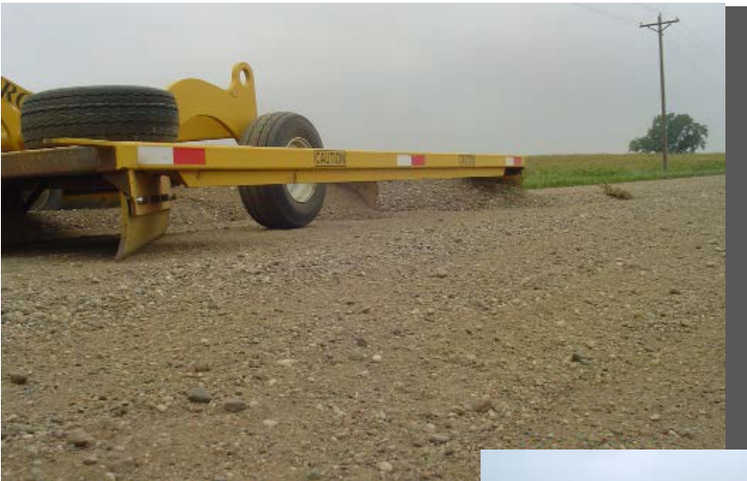
Example of a light blading device being towed by a mower tractor.
