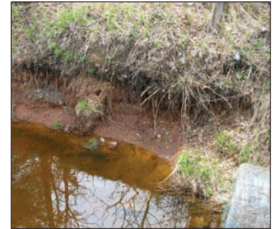
Figure 26: Side slope erosion (sloughing)
