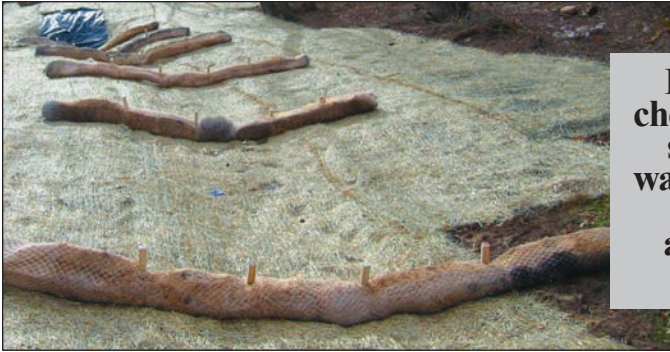
Figure 19: Bioroll check dam
