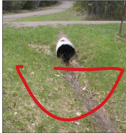
Figure 35: Example of a stable ditch shape
