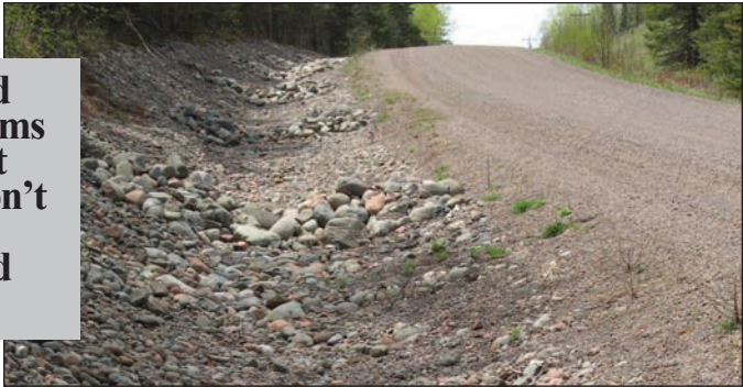
Figure 20: Rock check dam
