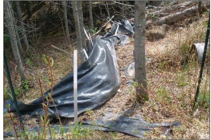
Figure 25: Remove silt fence when vegetation is established
