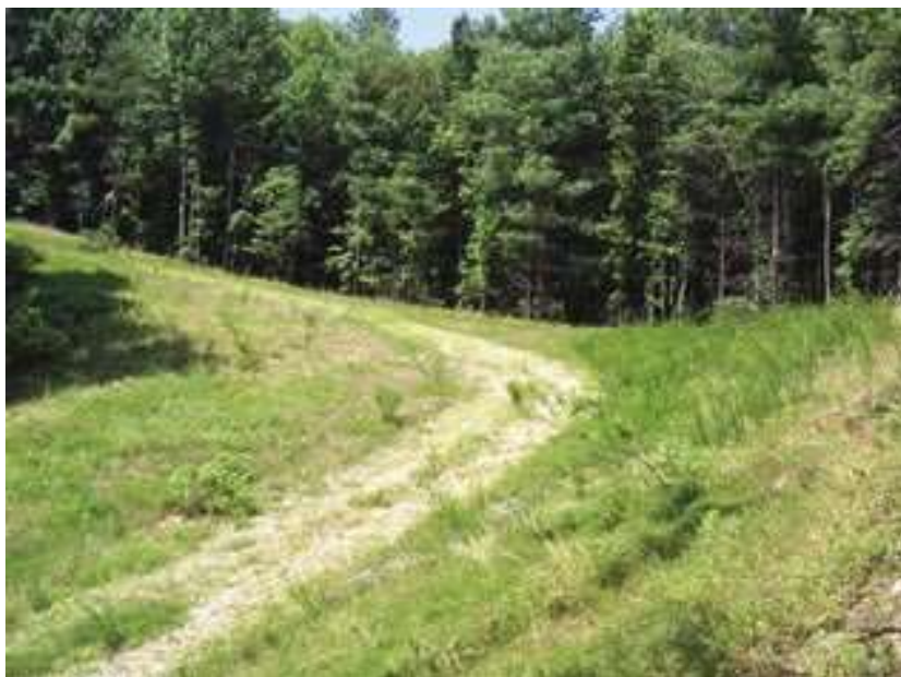
Stabilized forest access road. Note side/cut banks angled appropriately to minimize erosion.
