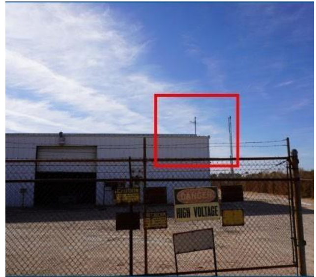
Figure 16. Light designed to illuminate when a dangerous concentration of H 2 S is detected. (Credit: CSB)
