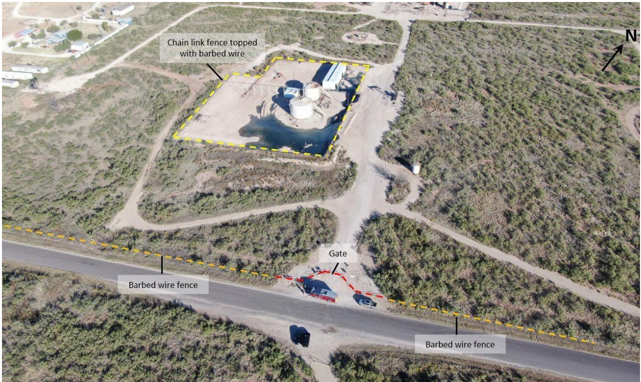
Figure 11. Aghorn waterflood station security. (Credit: CSB)
