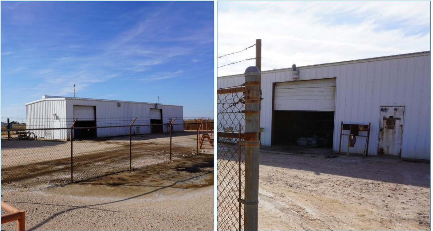
Figure 26. Photos showing bay door positions. (Credit: CSB)
