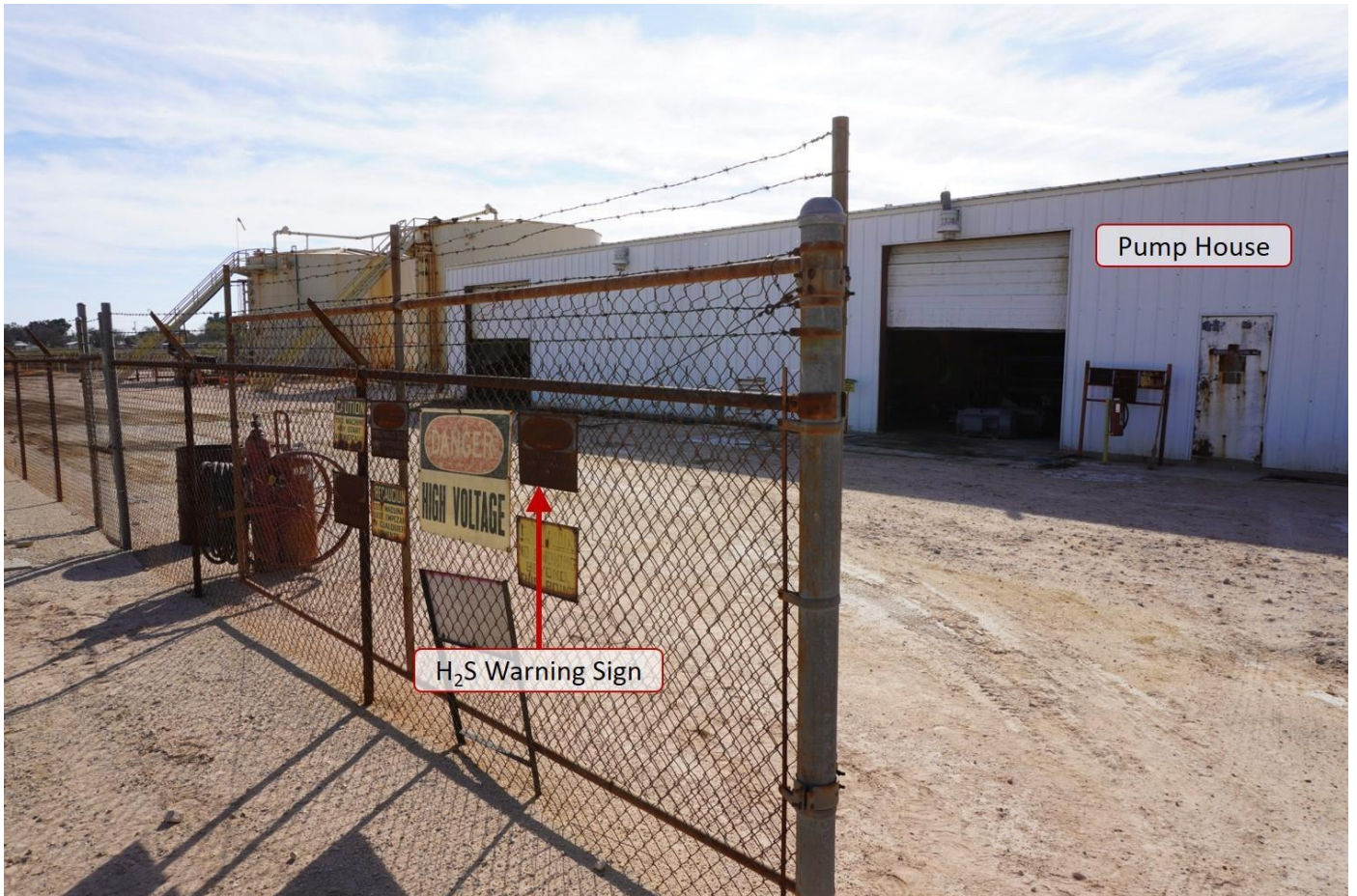
Figure 13. Warning signs and interior fence surrounding the waterflood station. (Credit: CSB)
