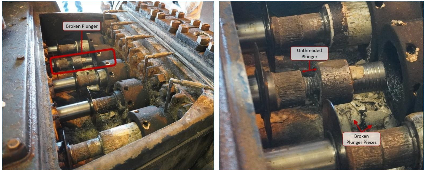
Figure 10. Photos of Pump #1 cradle and visible broken plunger pieces. (Credit: CSB)
