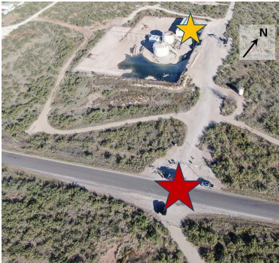
Figure 23. Location of the incident command post (red star) and incident location (gold star). (Credit: Ector County Sheriff’s Office)
