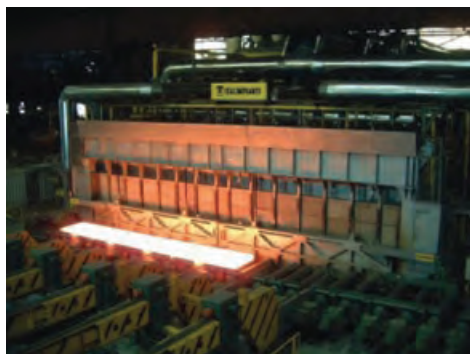
A walking beam furnace for metal reheating.
