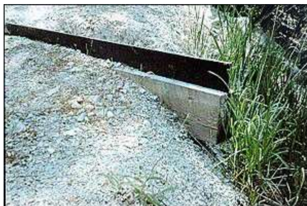
A deflector should be installed with approximately 3 inches of belting above the road surface.
