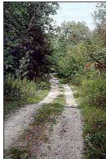
A drainage dip is effective in controlling water on the road and does not significantly slow the speed of vehicles.
