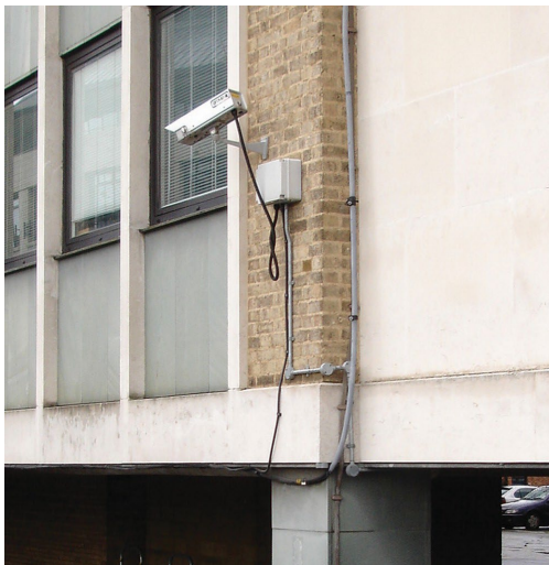
Figure 65. Conventional down-conductor separation distance problem.
