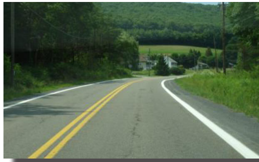
Roadway with 8-in edge line
