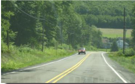
Roadway with 4-in edge line
