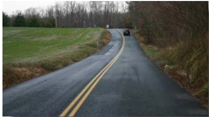
Centerline for No Passing on horizontal curve.
