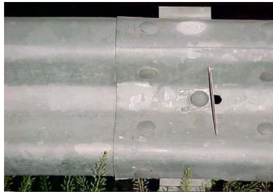
Installation of reflectors on W-beam guardrail.
