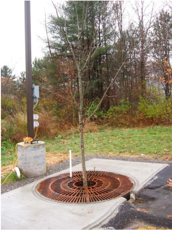
An example of a tree filter. (Source: University of New Hampshire Stormwater Center)
