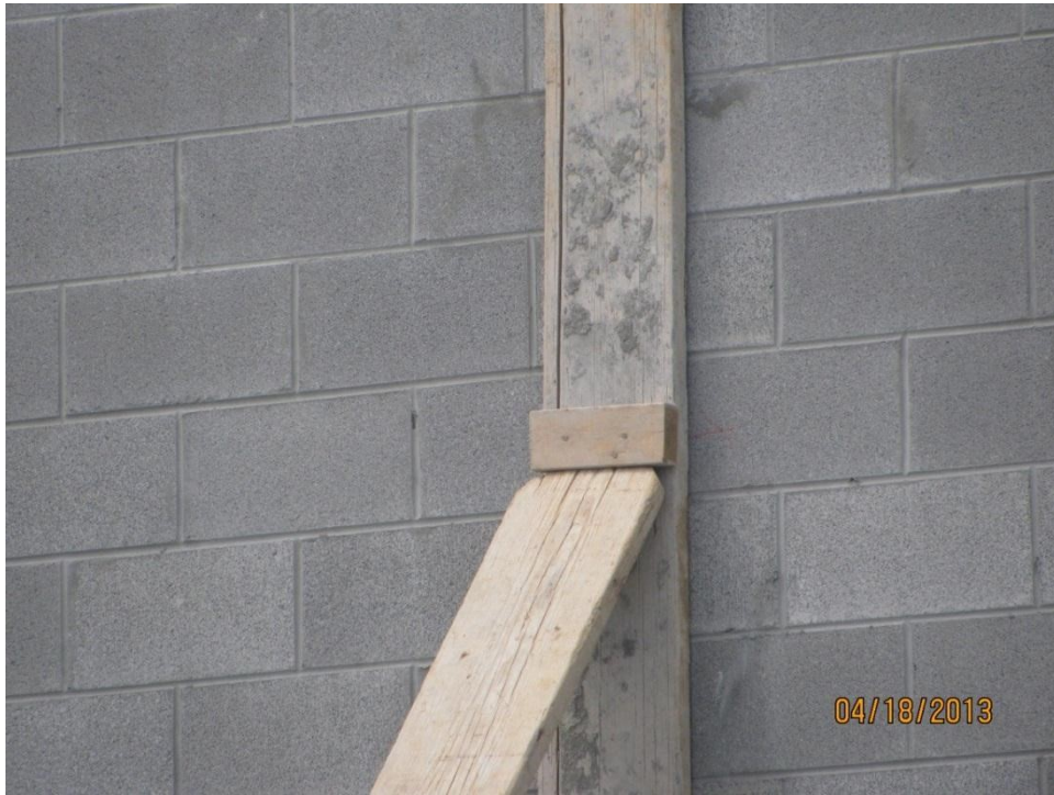
Figure 9 - Top end of brace without positive connection
