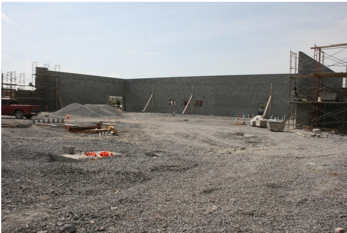
Figure 6 – Typical interior bracing detail
