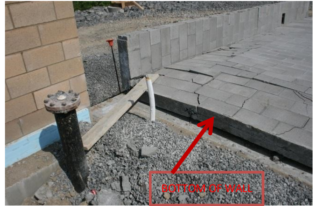
Figure 21 - Collapsed wall
