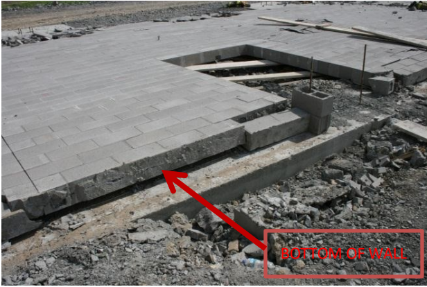
Figure 19 - Collapsed wall
