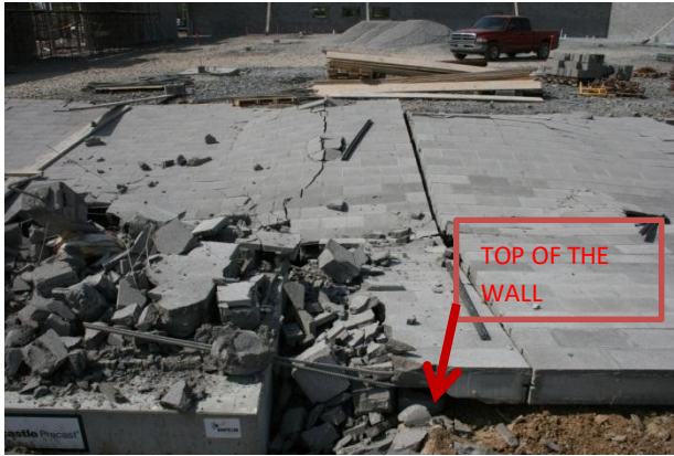
Figure 20 - Collapsed wall Structural Analysis and Discussion
