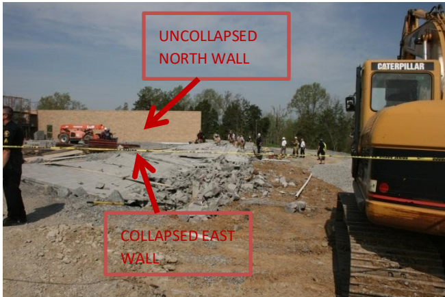
Figure 16 - Collapsed wall
