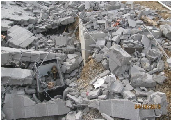
Figure 18 - Collapsed wall
