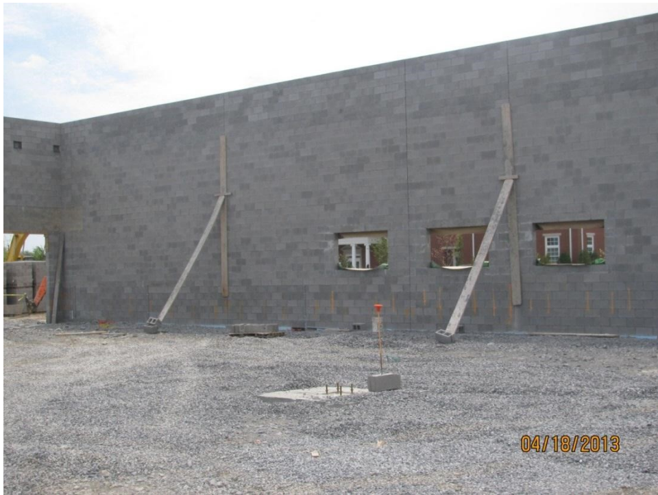
Figure 9 - Top end of brace without positive connection
