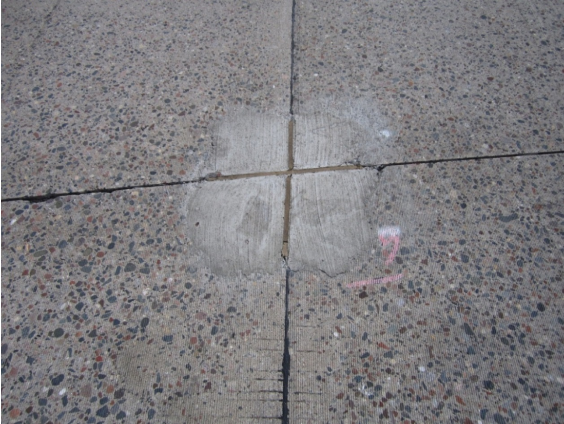
Figure 1.4. Typical MnROAD partial-depth repair with cementitious-based material.
