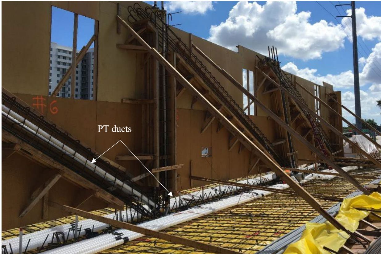
Figure 12 Main span deck longitudinal tendon ducts (Photo by BPA, date unknown)
