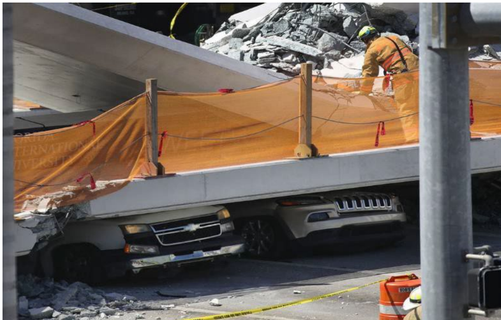
Figure 75 Vehicles crushed by falling bridge
