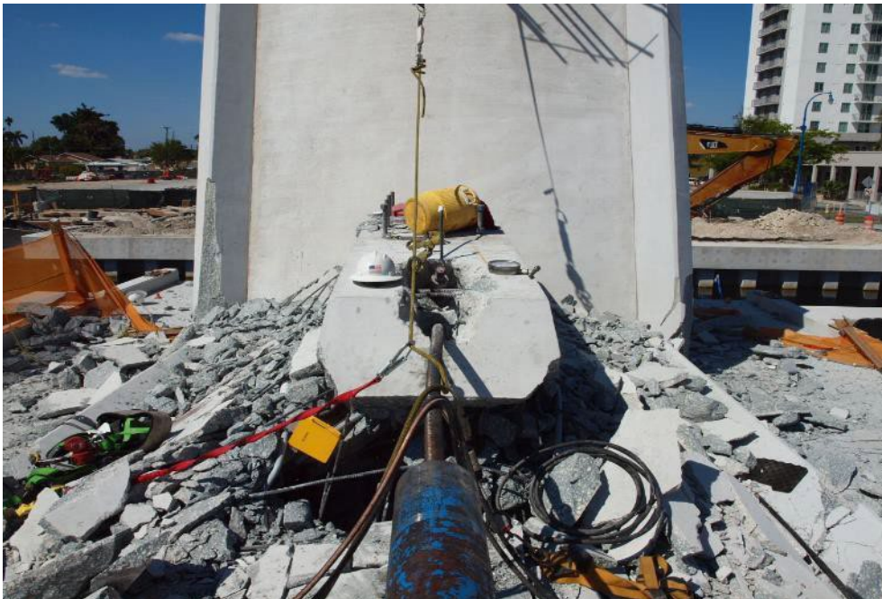
Figure 53 Northernmost blister and hydraulic jack attached to the lower PT bar of diagonal 11 after bridge collapse – side view, March 17, 2018 by OSHA
