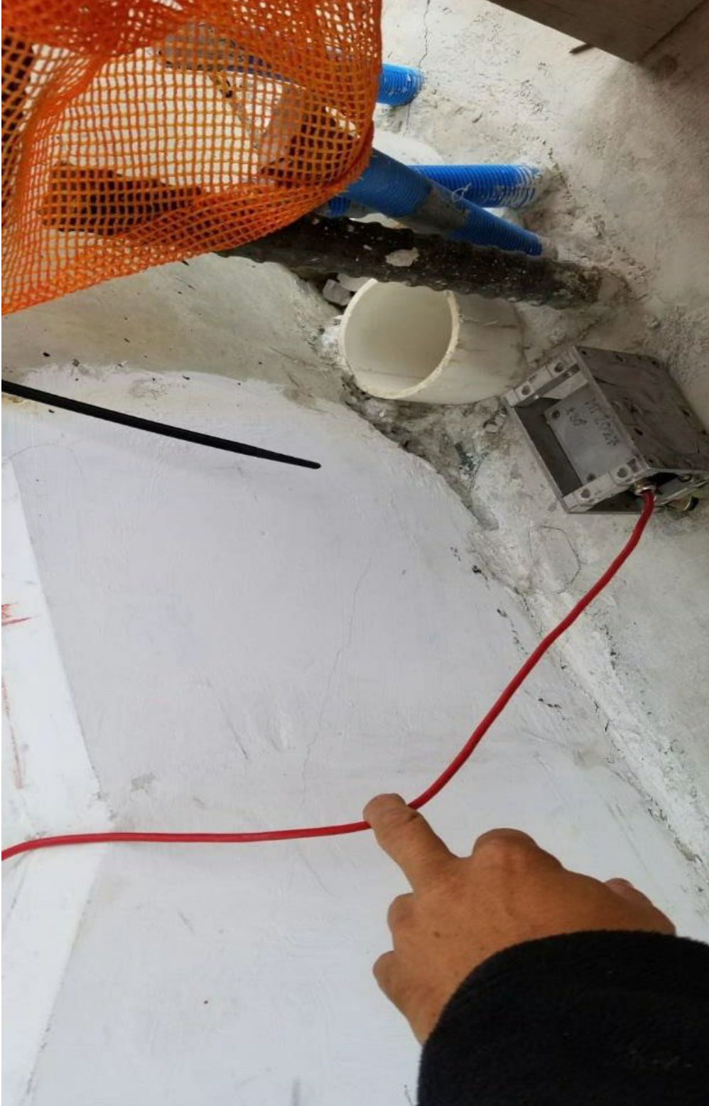
Figure 43 Cracks at the east side diaphragm II on 3/10/2018 – top face, by Corradino
