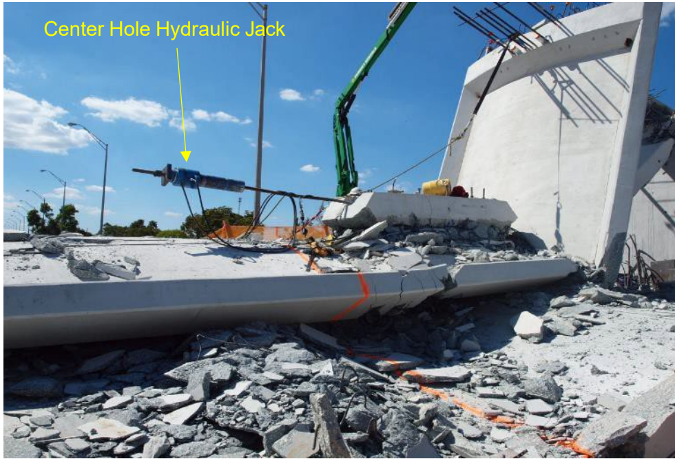
Figure 53 Northernmost blister and hydraulic jack attached to the lower PT bar of diagonal 11 after bridge collapse – side view, March 17, 2018 by OSHA
