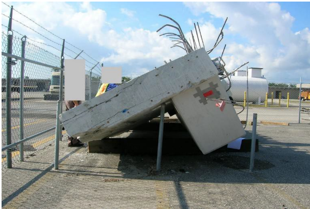
Figure 71 Side view of the saved portion of the diaphragm II in storage yard, April 9, 2018, by OSHA
