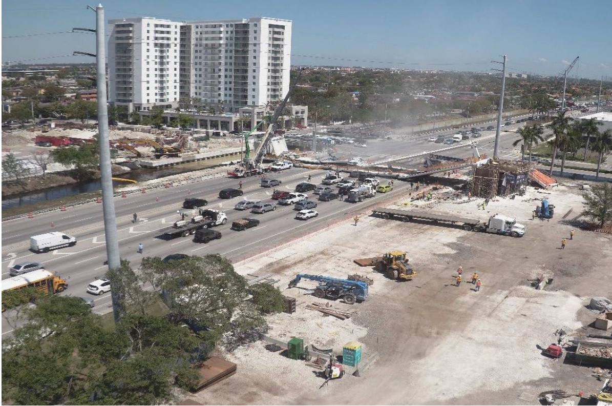
Figure 51 Bridge immediately after the collapse, March 15, 2018 – camera #3 (north on the left and south on the right)
