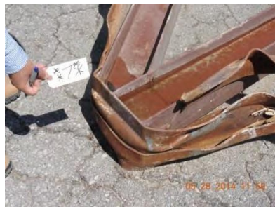
Fig. 42 – Joint 7 – East truss
