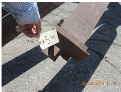
Fig. 20 – Joint 5 – North truss
