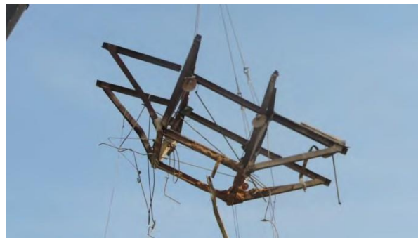
Fig. 105 Interior trusses being retrieved
