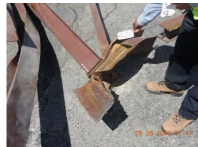
Fig. 36 – Joint 2 – East truss
