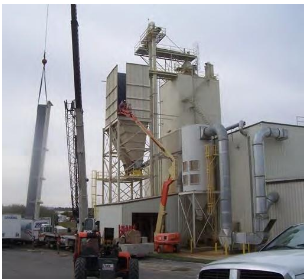
Fig. 7 Two outside bins being added
