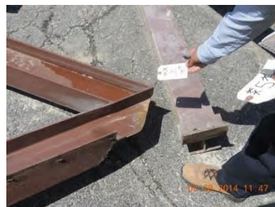
Fig. 38 – Joint 4 – East truss
