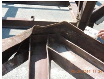
Fig. 21 – Joint 6 – North truss
