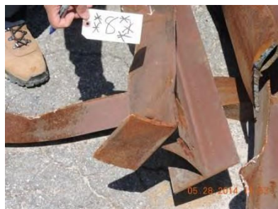
Fig. 51 – Joint 8 – West truss
