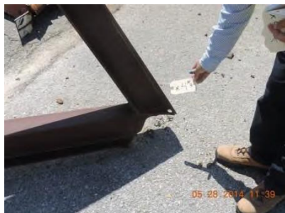
Fig. 28 – Joint 4 – South truss
