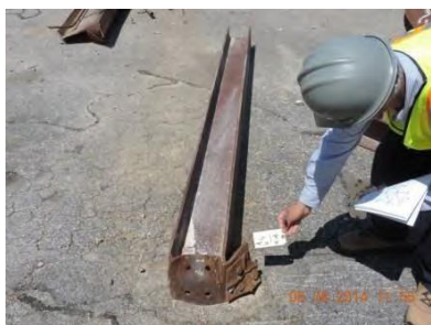
Fig. 44 – Joint 1 – West truss
