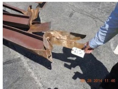
Fig. 35 – Joint 1 – East truss
