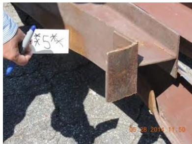
Fig. 40 – Joint 5 – East truss
