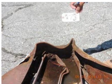
Fig. 50 – Joint 7 – West truss
