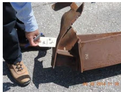
Fig. 24 – Joint 1 – South truss
