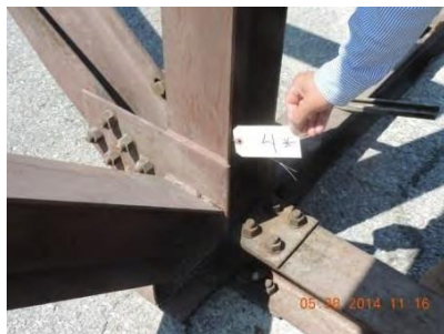
Fig. 55 – Joint 4 – East interior
