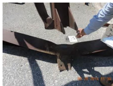
Fig. 27 – Joint 3 – South truss
