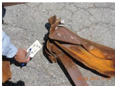
Fig. 45 – Joint 2 – West truss
