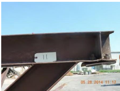
Fig. 76 – Joint 11 – South interior
