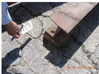
Fig. 43 – Joint 8 – East truss
