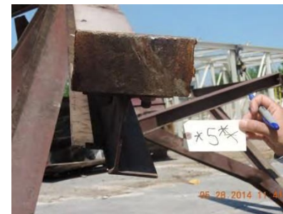
Fig. 30 – Joint 5 – South truss
