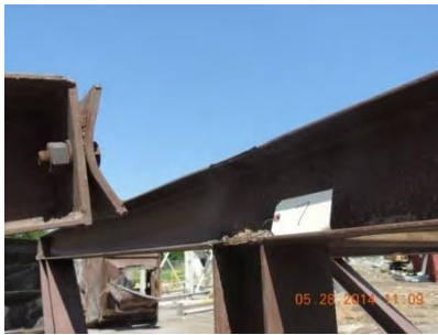
Fig. 70 – Joint 7 – South interior
