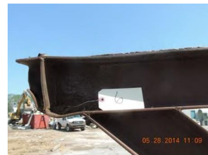
Fig. 69 – Joint 6 – North interior
