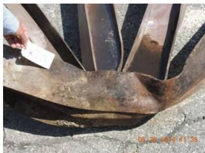
Fig. 22 – Joint 7 – North truss
