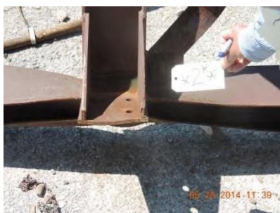
Fig. 26 – Joint 2 – South truss
