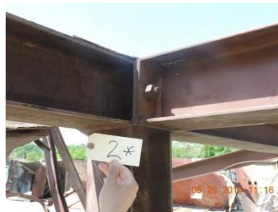
Fig. 53 – Joint 2 – East interior
