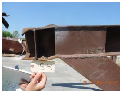
Fig. 56 – Joint 5 – East interior
