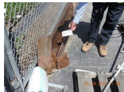
Fig. 39 – Joint 4 – East truss
