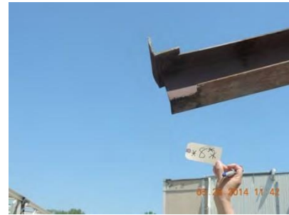
Fig. 33 – Joint 8 – South truss
