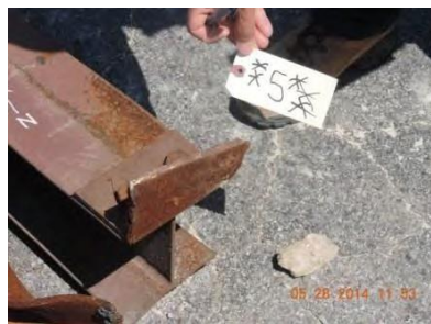
Fig. 48 – Joint 5 – West truss
