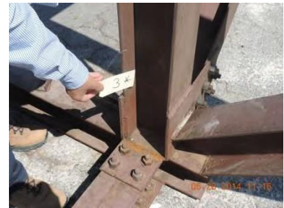
Fig. 54 – Joint 3 – East interior
