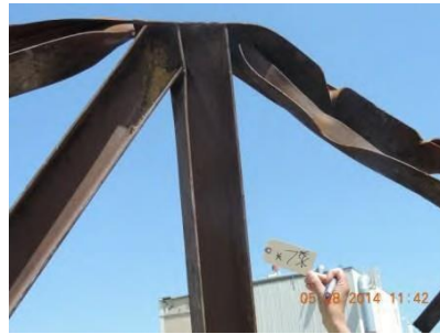
Fig. 32 – Joint 7 – South truss
