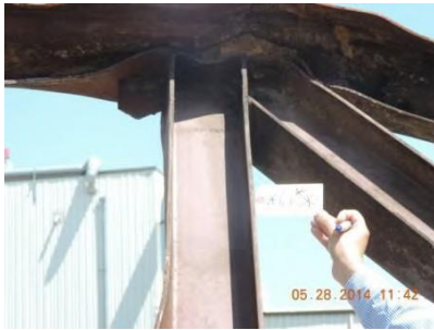
Fig. 31 – Joint 6 – South truss
