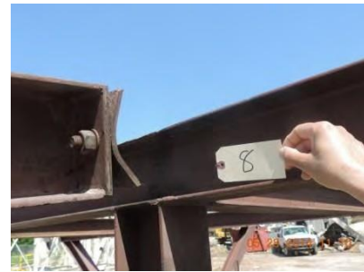
Fig. 72 – Joint 8 – South interior
