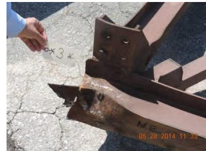
Fig. 18 – Joint 3 – North truss
