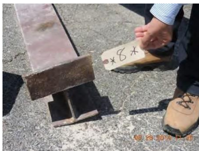
Fig. 23 – Joint 8 – North truss
