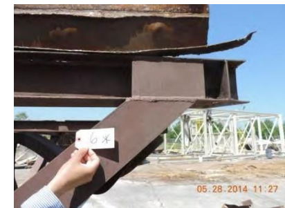
Fig. 57 – Joint 6 – East interior
