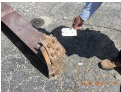
Fig. 34 – Joint 1 – East truss
