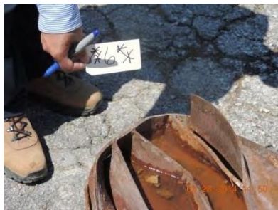
Fig. 41 – Joint 6 – East truss
