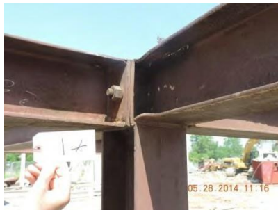
Fig. 52 – Joint 1 – East interior
