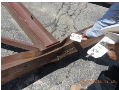
Fig. 37 – Joint 3 – East truss
