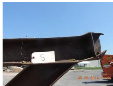
Fig. 68 – Joint 5 – North interior
