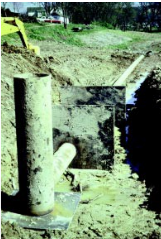
Figure 22 Drop-inlet pipe spillway with antiseep collar
