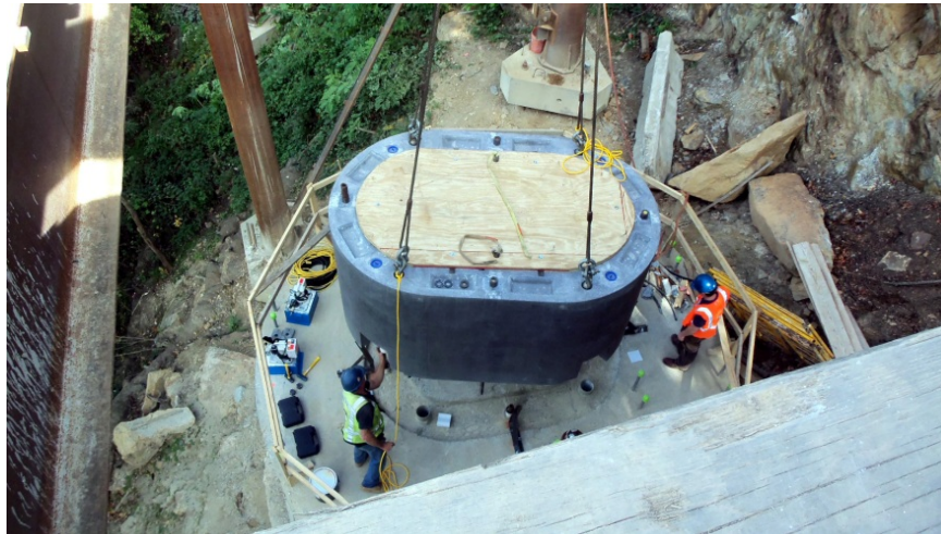
Figure 1.32 - Precast Hollow Segmental Piers, Foothills Bridge No. 2
