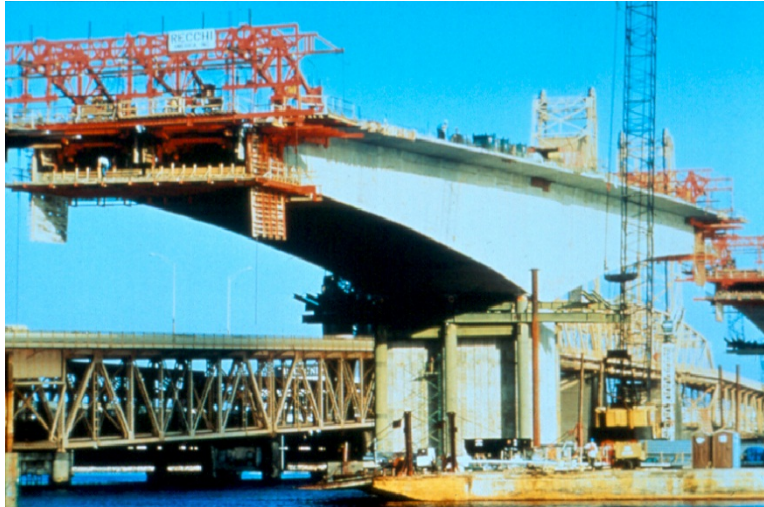
Figure 1.17 - Cast-In-Place Segmental Construction using Form Travelers
