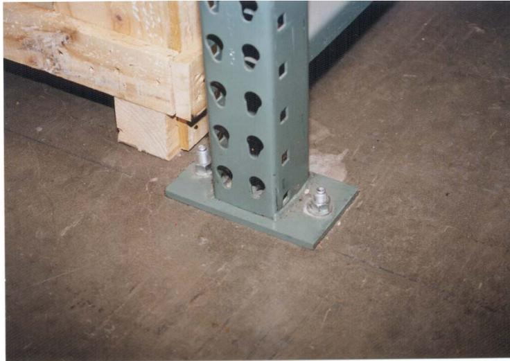
*Figure 1-5 Typical column base plate connection.*
