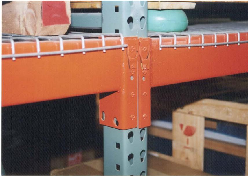
*Figure 1-3 Typical proprietary moment connection.*
