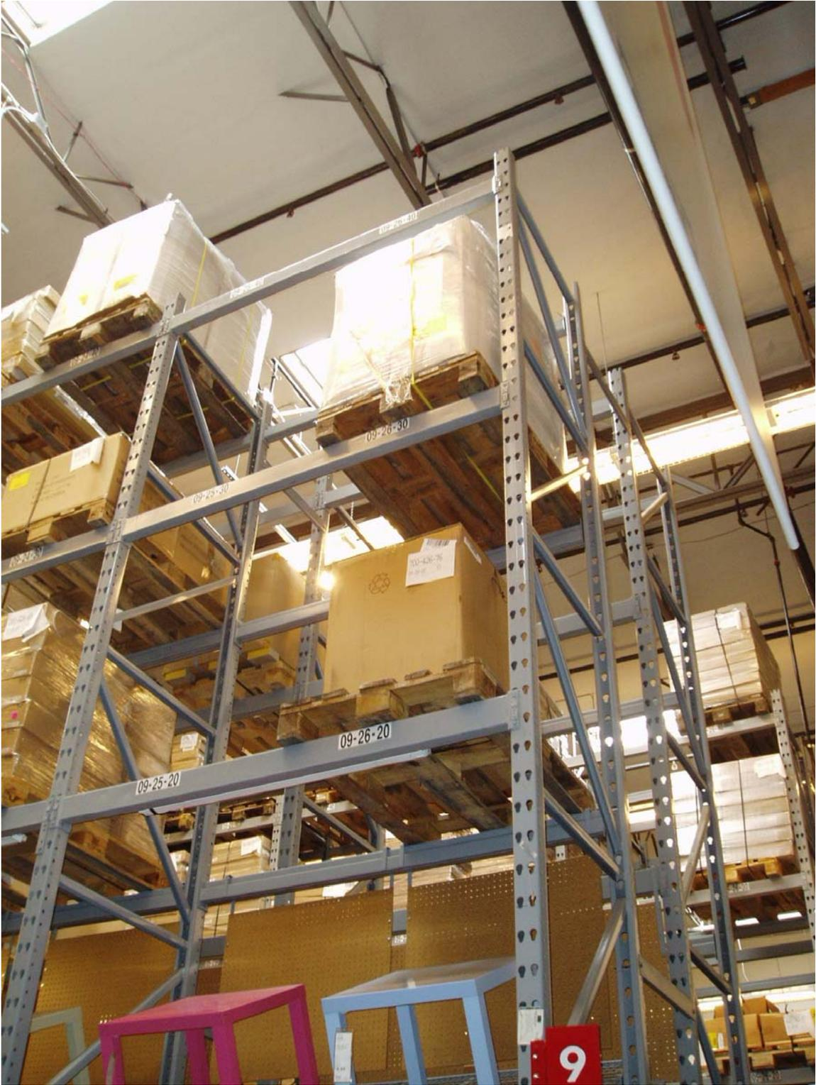
*Figure 8-2 Pallets in this home furnishings store are supported only on the beams and may slide off these supports during an earthquake.*
