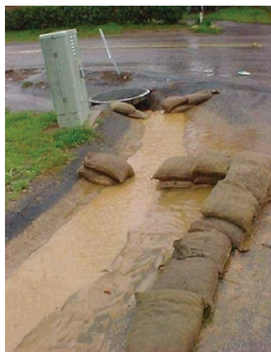
Figure 5. Make sure storm drain inlets are protected.
