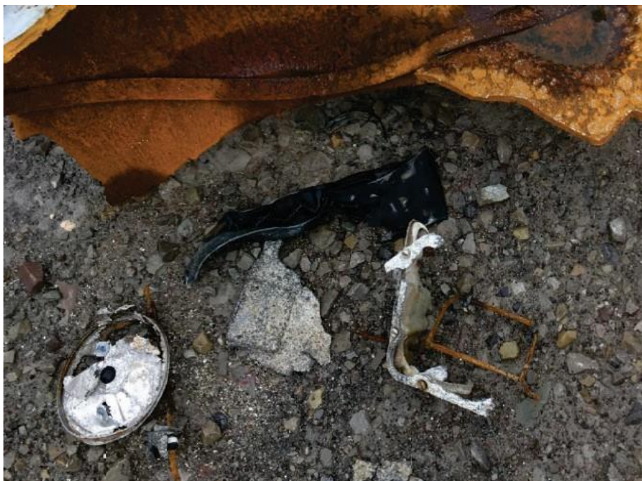
Figure 13. Aluminum Parts. This photo shows aluminum internal components that were likely in the middle chamber of the MP odorizer, found after the May 24, 2017, incident. The explosion destroyed the aluminum pan and components that were inside the middle chamber of the MP odorizer. (Credit: SPSI).
