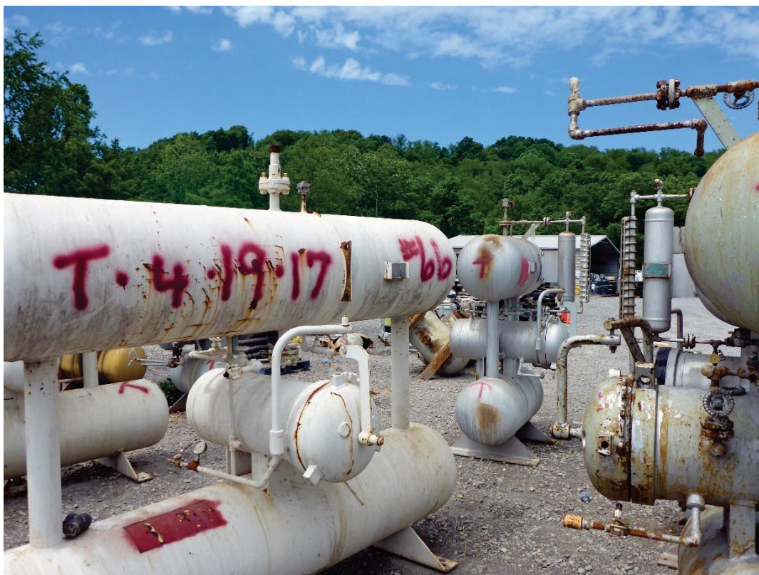
Figure 7. Treatment Status. This photo shows how MRR technicians used red spray paint to record the date the MP was chemically treated, April 19, 2017. (Credit: CSB).
