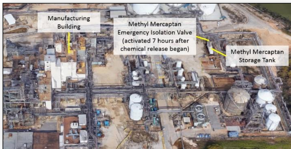
Figure 13. Location of Methyl Mercaptan Emergency Isolation Valve Relative to Manufacturing Building Where Leak Occurred. The emergency isolation valve was not activated until seven hours after the release began. Source: Google Earth, with annotations by CSB.
