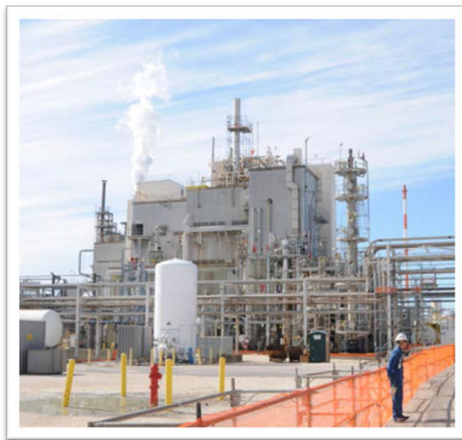
Figure 1. The Lannate ® Manufacturing Building. The methyl mercaptan release occurred in the manufacturing building. Source: CSB.
