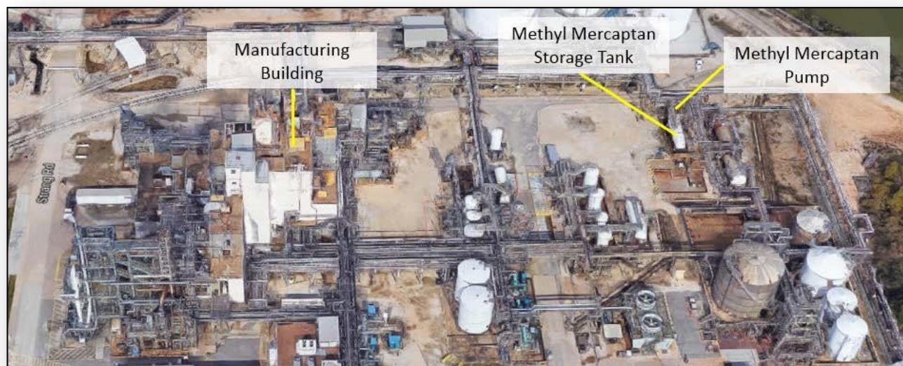
Figure 7. Location of Methyl Mercaptan Pump. The pump was turned off nearly three hours after the release began. Source: Google Earth, with annotations by CSB.
